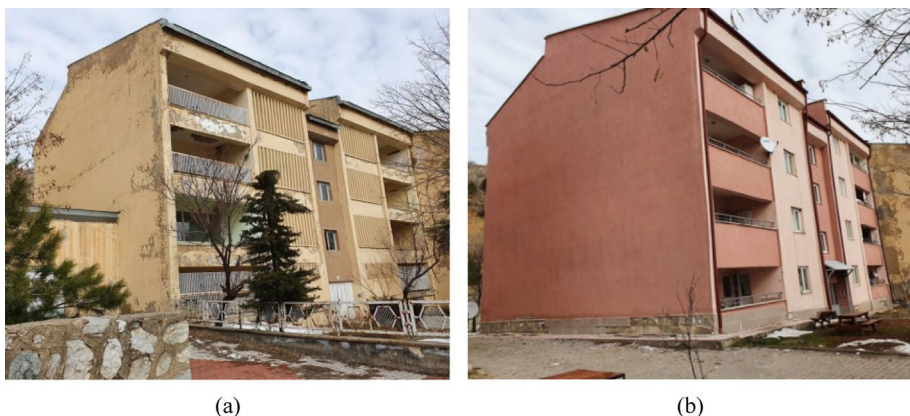
Fig. 3 Investigated buildings a non-retrofitted b retrofitted
