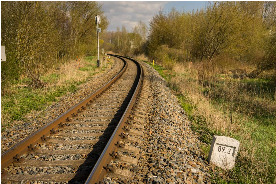
Image 15 - left leaning curve on the 237 line, which would form a part of the proposed triangular junction, with a distance marker on the right.
