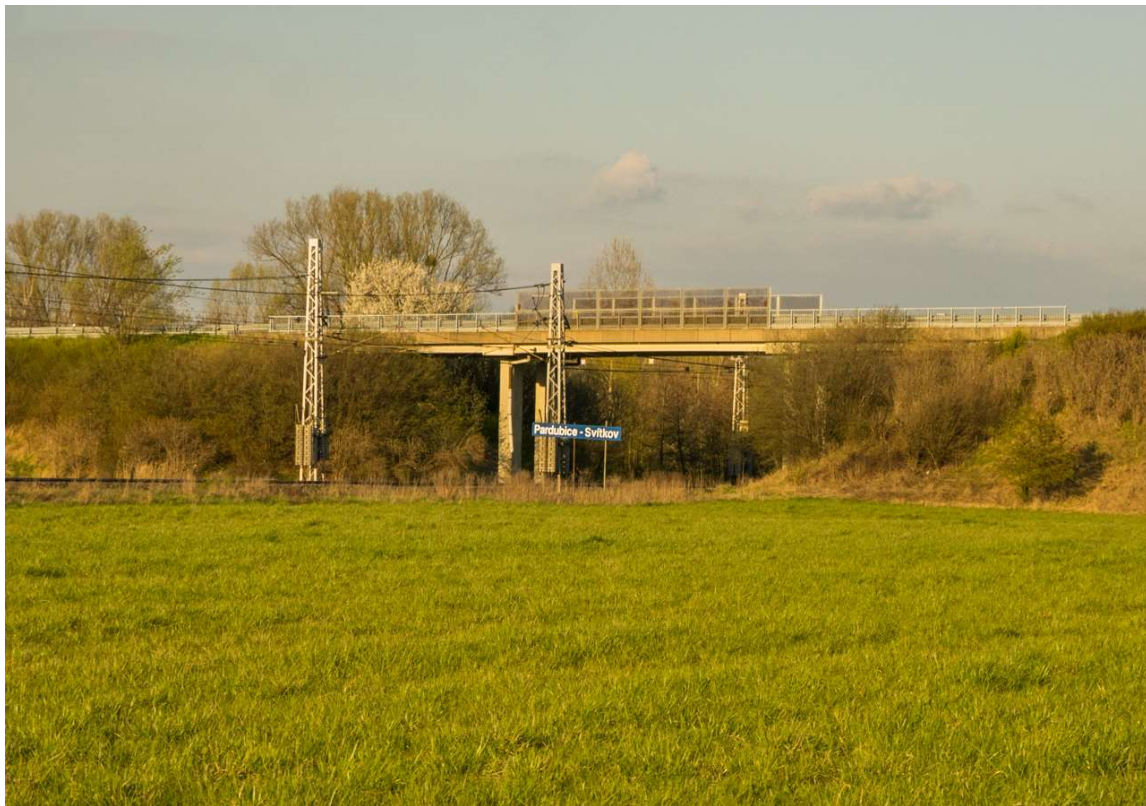
Image 35 - a road beam bridge east of the proposed triangular junction of the variant C line, located near the Pardubice Svítkov railway halt.
