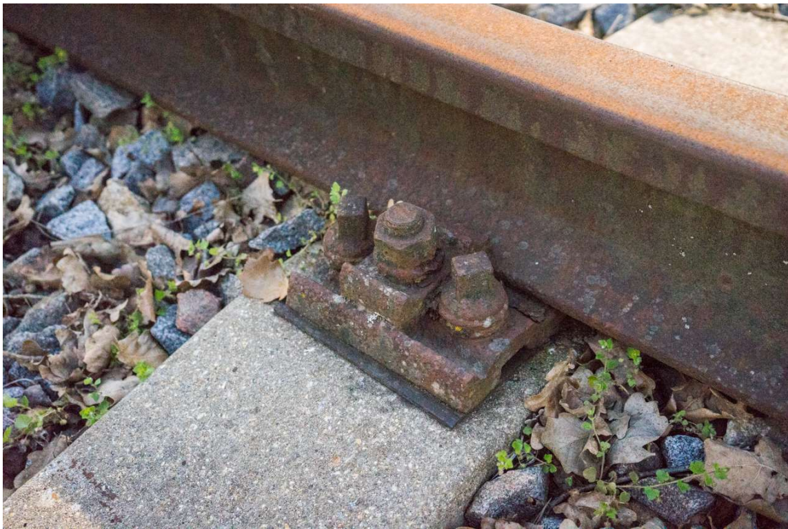
Image 6 - detailed view of the branch line fastener and the concrete ballast
