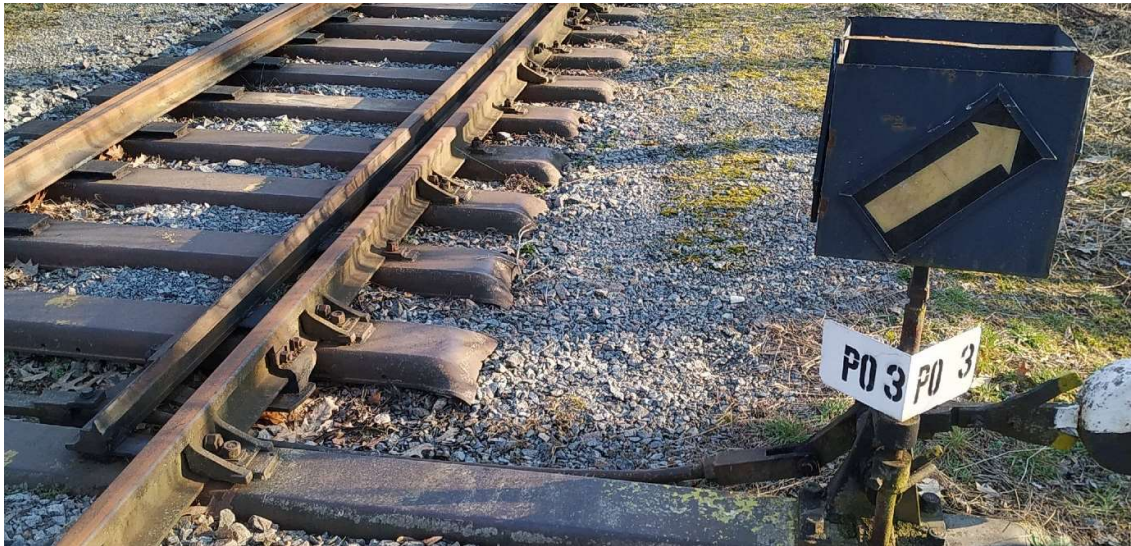
Figure 22 - rail switch located outside the compound, dividing the branch line into a tangent side-track and right handed curve inside the airport compound.
