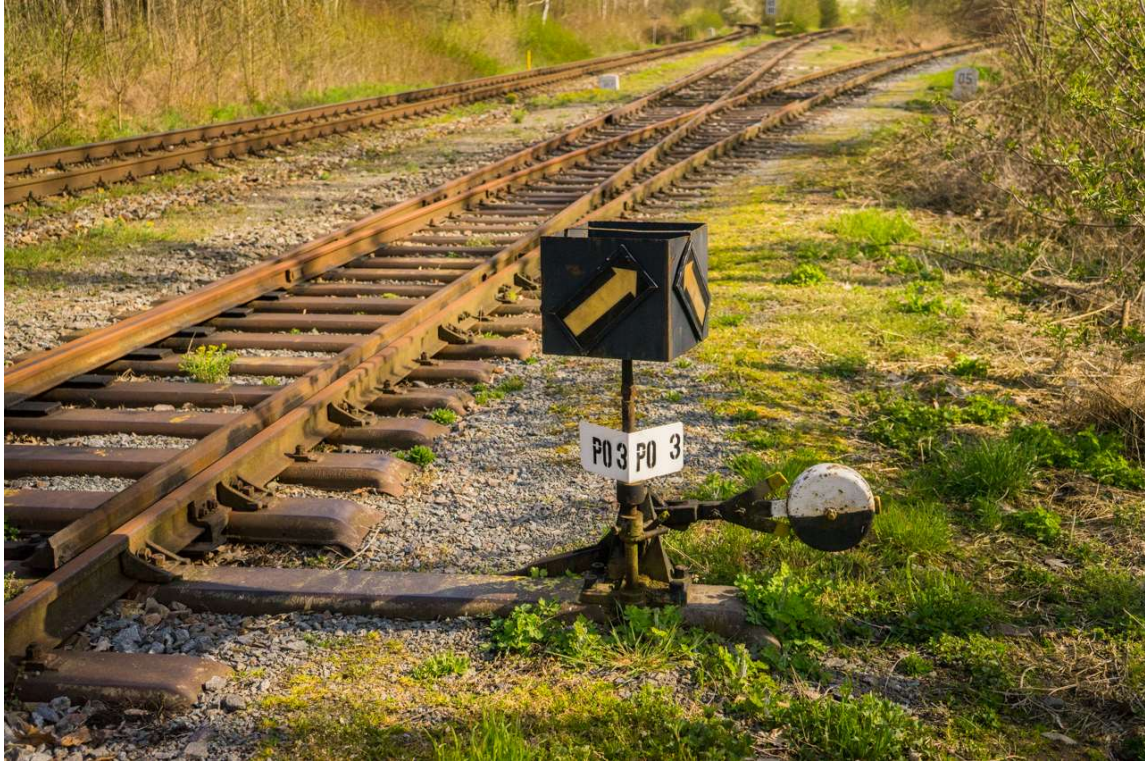
Image 7 - railroad switch located on the edge of the airport compound separating the branch line into a tangent side-track with the main track curving right into the eastern portion of the airport compound.
