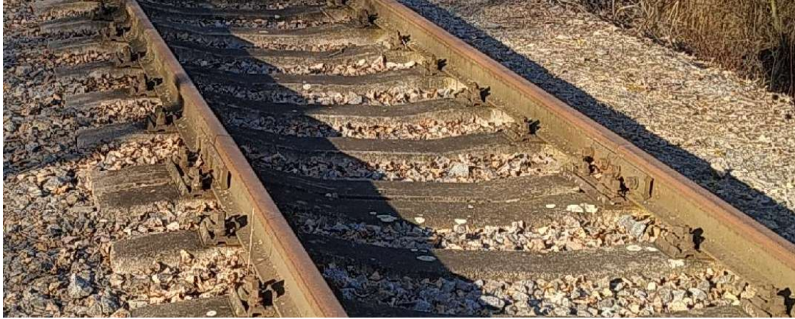
Figure 21 - a portion of the track on the main branch line with rail joints.
