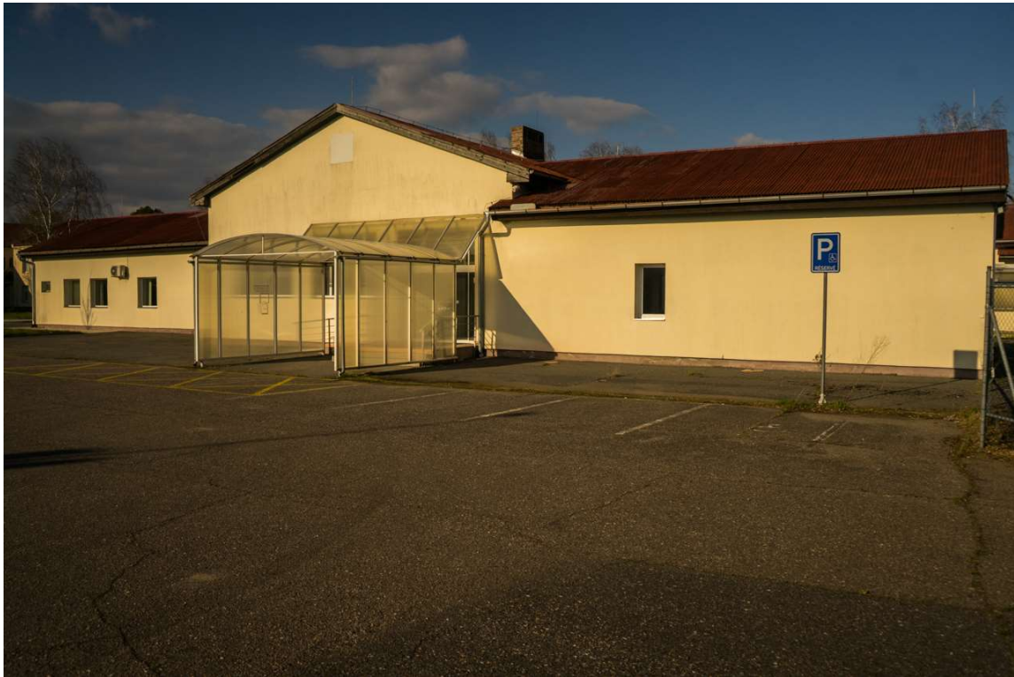
Image 29 - view of the old airport terminal building
