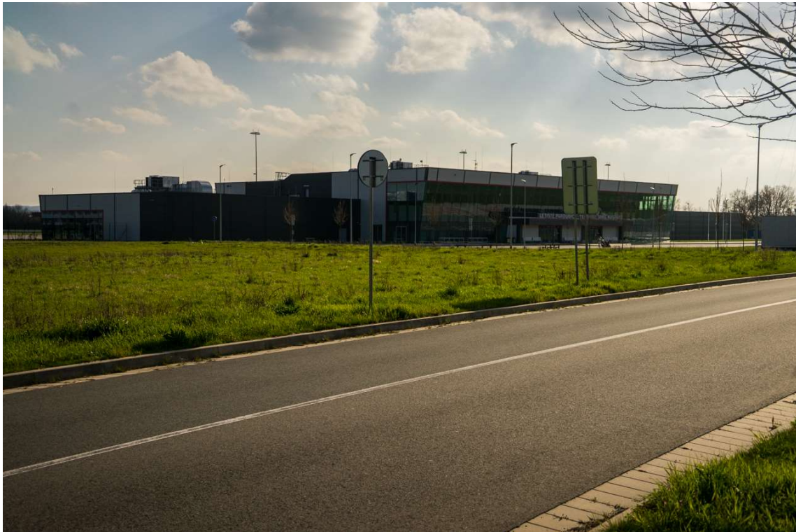
Image 17 - View of the Jan Kašpar Terminal with the site of the proposed railway station in A and B variants in the front
