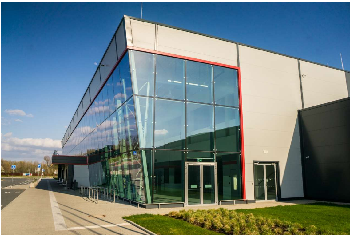
Image 22 - Jan Kašpar airport terminal main hall viewed from its western side for reference.
