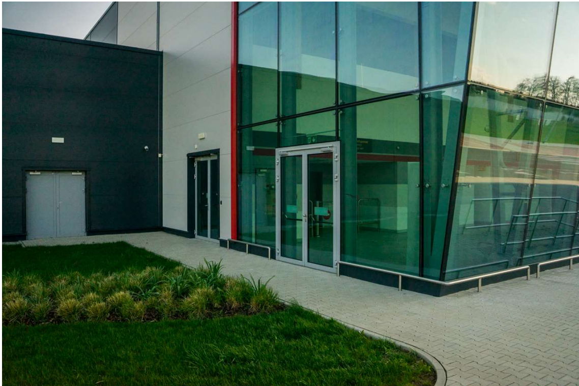
Image 21 - site of a possible entrance of the passageway of the variant B to the Jan Kašpar terminal, an emergency exit door utilized as an entrance to the passageway.
