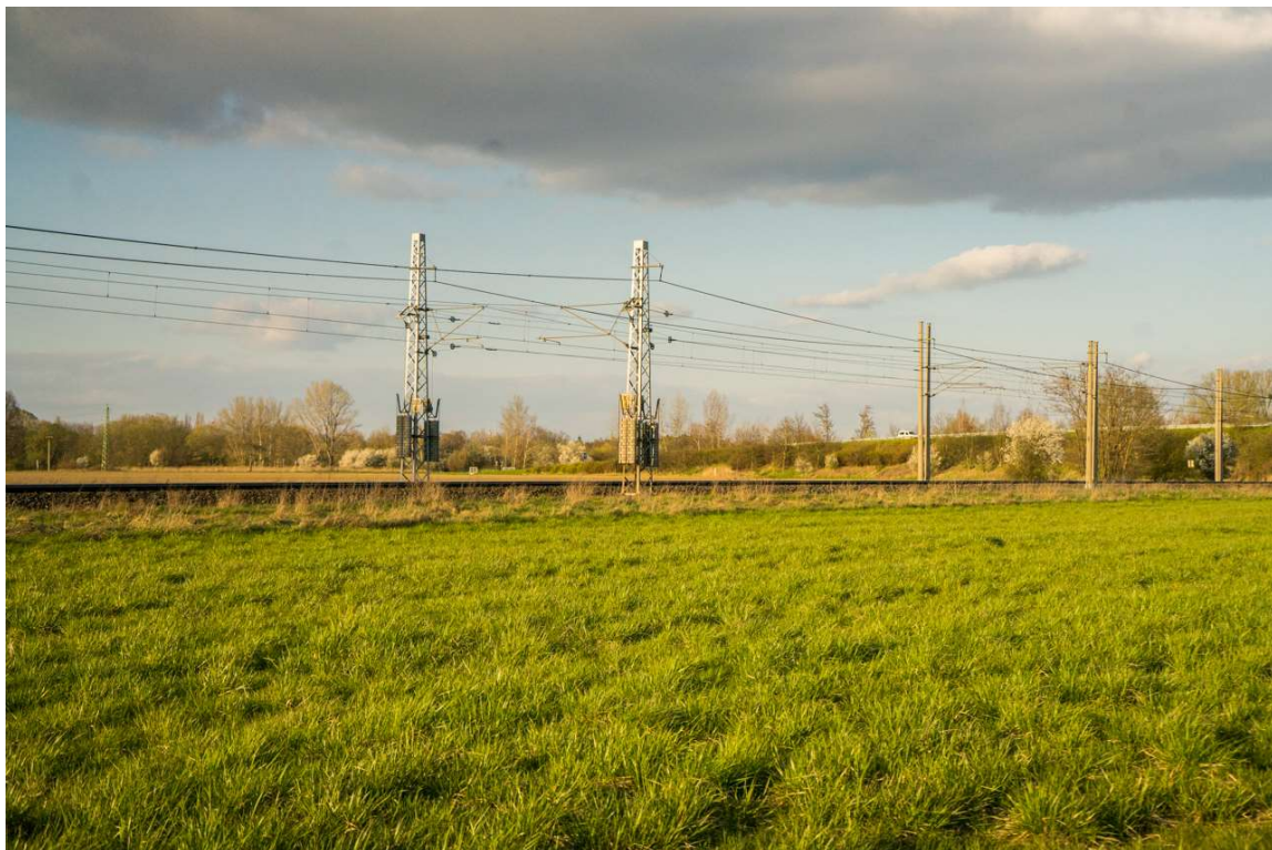
Image 36 - view of the first and third corridor line, where the variant C would connect to the railway network.
