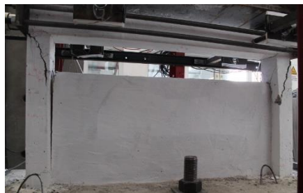
Fig. 2. Excessive shear cracks on the captive columns before repairing (CFRPE_02)
