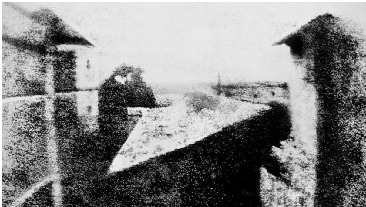
Obrázek 2 - Pohled z okna v Le Gras (Zdroj: Rebecca A. Moss, Coordinator of Visual Resources and Digital Content Library, via email. College of Liberal Arts Office of Information Technology, University of Minnesota. http://www.dcl.umn.edu )
