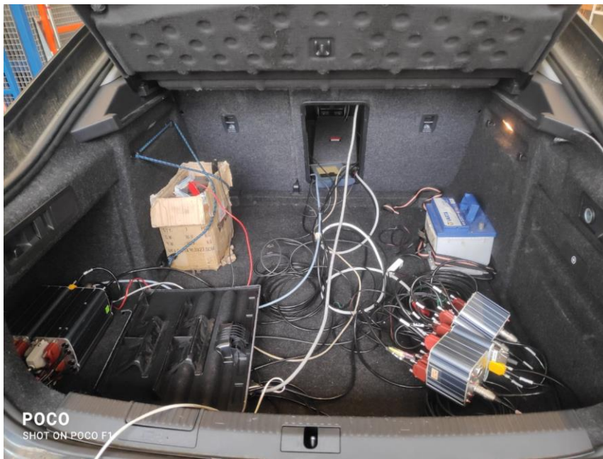
Figure 9– The control panel including the batteries
