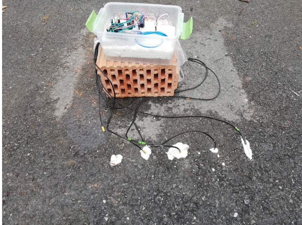
Figure 22 Thermometer sensors installed in the site number 2, semi-rigid pavement
