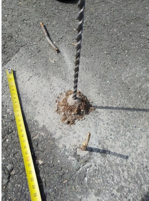
Figure 16 The drilling steps in the site
