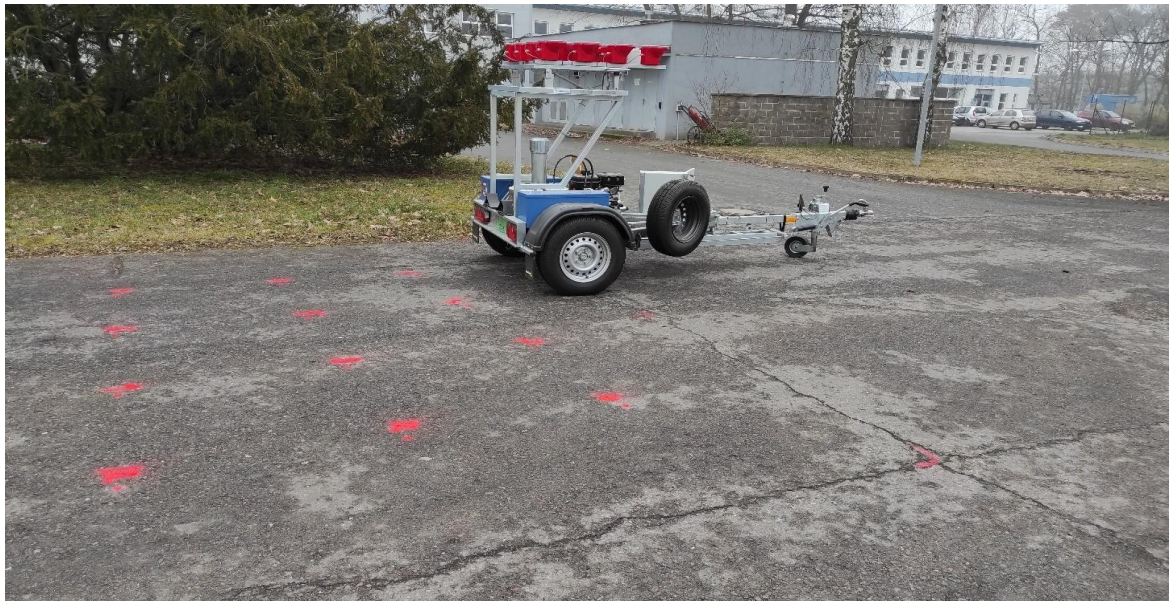
Figure 20 Preparation for the site number two, semi-rigid pavement
