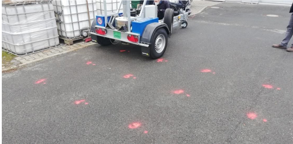
Figure 17 Preparation site number number1, flexible pavement.
