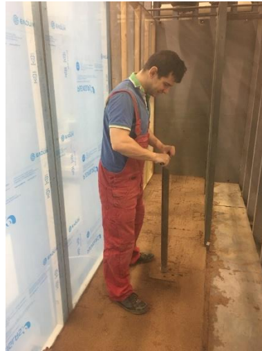
Figure 6.2 Preparation of foundation layer
