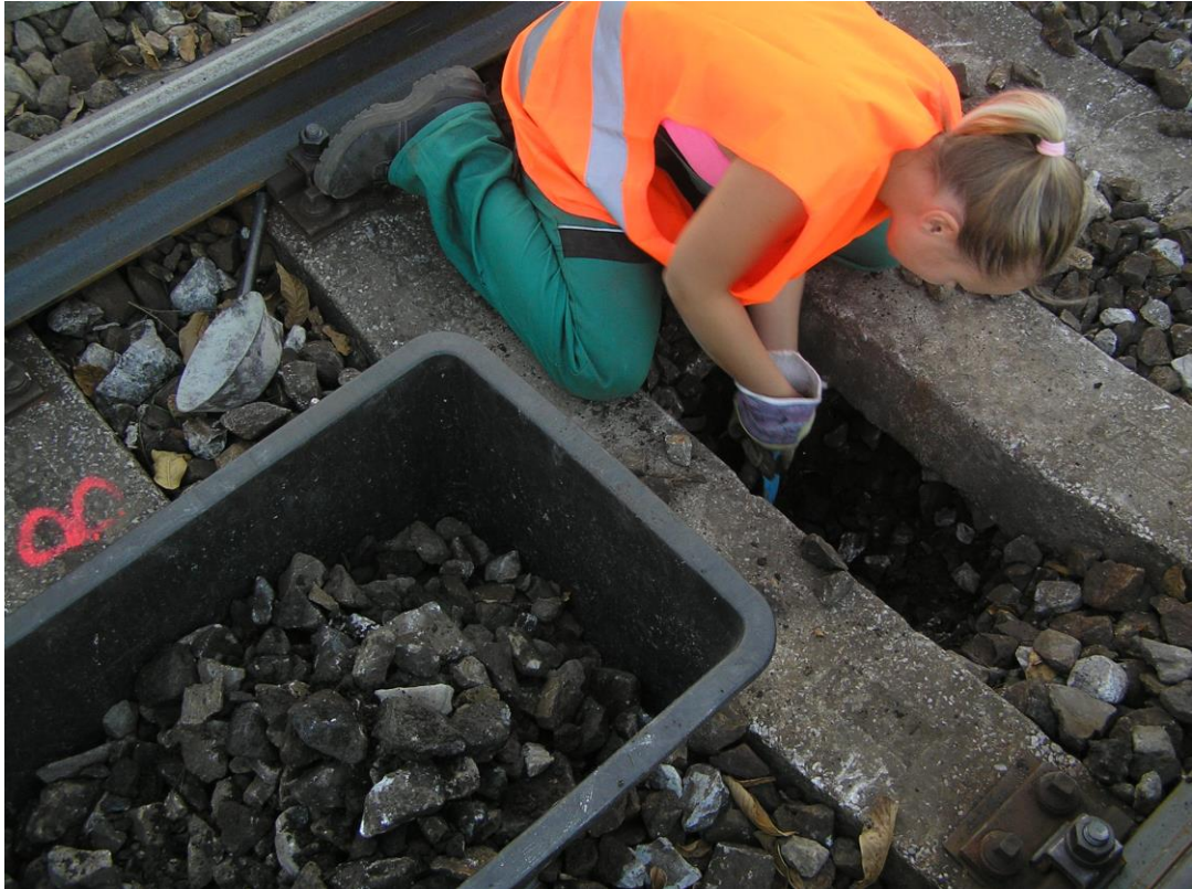
Figure 35 – Excavating of the probe 2 material (P2U2)
