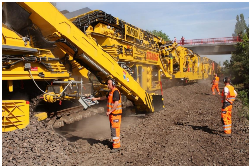
Figure 2 – RM 900 VB used on railway track section Kutná Hora – Čáslav [2]
