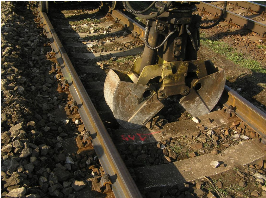
Figure 34 – Extracting of the probe 1 material (P6U1)
