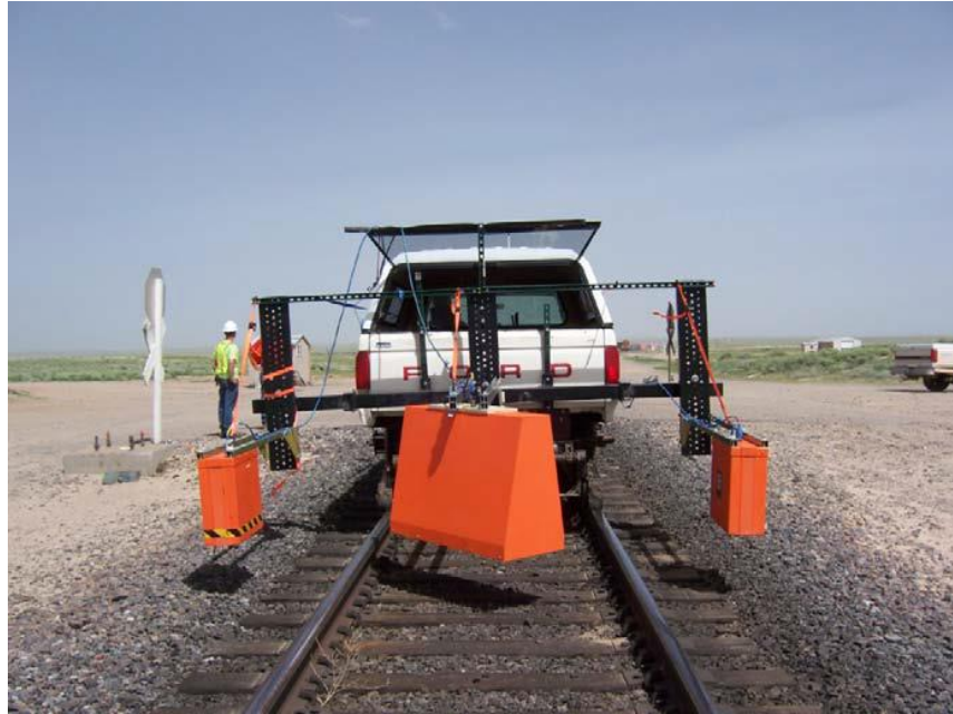
Figure 12 - GPR equipment on railroad track using two 2GHz antenna and one 500MHz antenna. [34]
