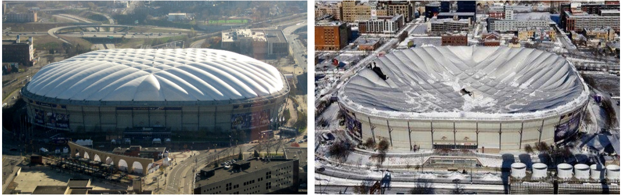
Figure 2.5. Failure of the Metrodome’s roof arising from the weight of snow and ice [36].
