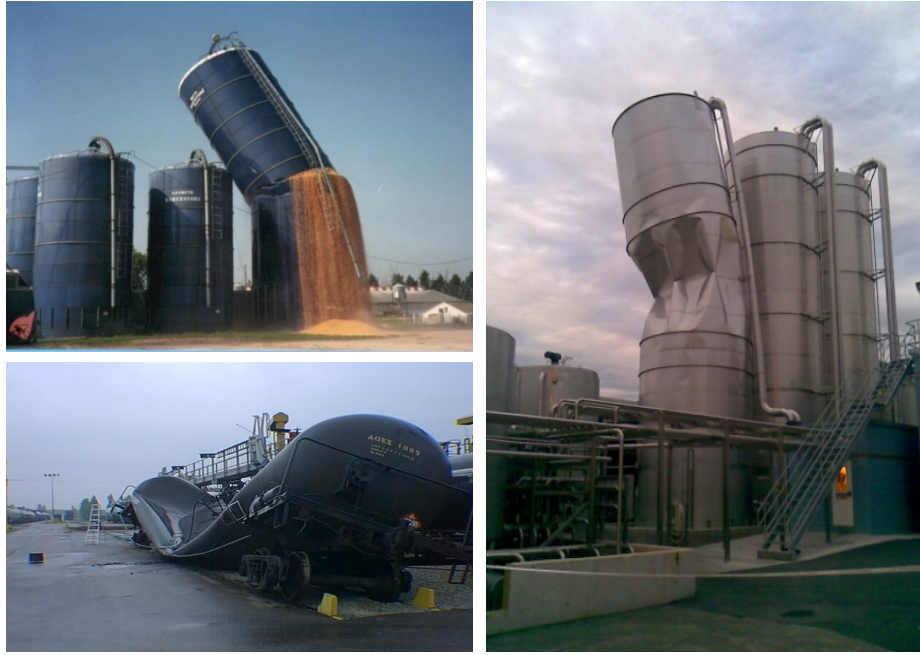
Figure 2.4. Failure examples caused by loss of stability in practice [33, 34 and 35].
