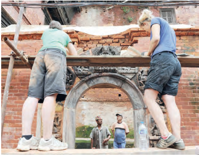
Fig. 10 Patan, reassembling of the stone gates. (Institute of Conservation, University of Applied Arts Vienna, 2012)
