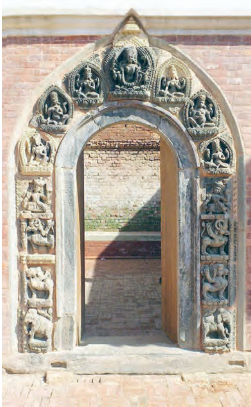
Fig. 19 Patan, Stone Gates after the treatment in 2012, new and old parts are very different in color. (Institute of Conservation, University of Applied Arts Vienna, 2013)
