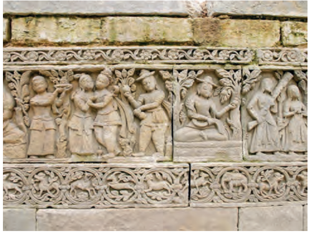
Fig. 3 Patan, Bhandarkhal Tank Pavilion, carving spreads regardless of the joint net. (Institute of Conservation, University of Applied Arts Vienna, 2010)
