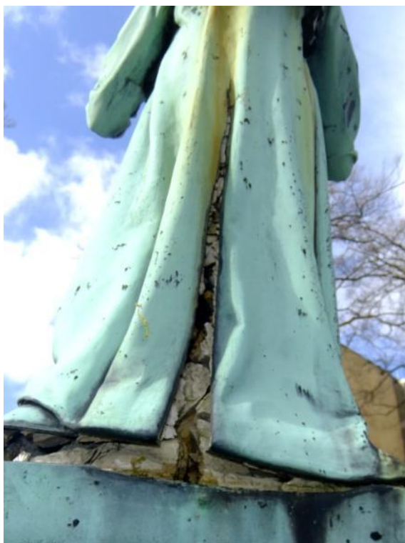
Obr. III. /45. Hrob rodiny Ratschky, detail praskliny na galvanoplastice.
