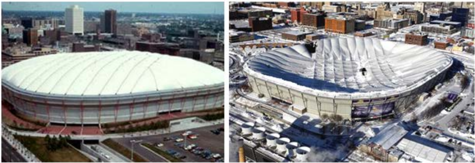
Fig. 4 Roof of the stadium in Minneapolis
