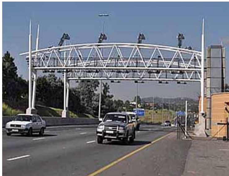
Figure 21: Open road tolling
