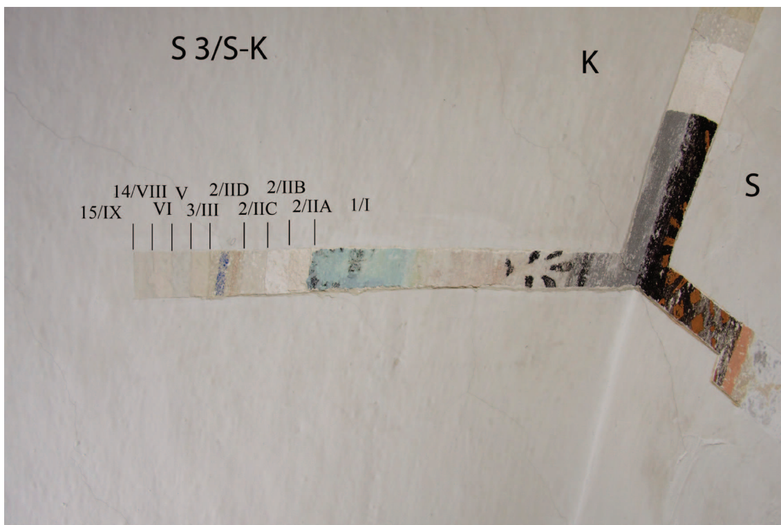
Obr. 19: Sonda S 3/S-K, klenba, detail.
