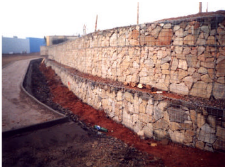
Obr. 2 Opì mážeì z dráokoš ù– gabionù Fig. 2 Abutment wall from wire-scrapes - gabions
