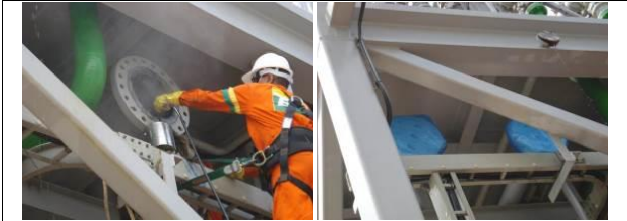
Figure 72 – Oil & Gas – Internal protection
