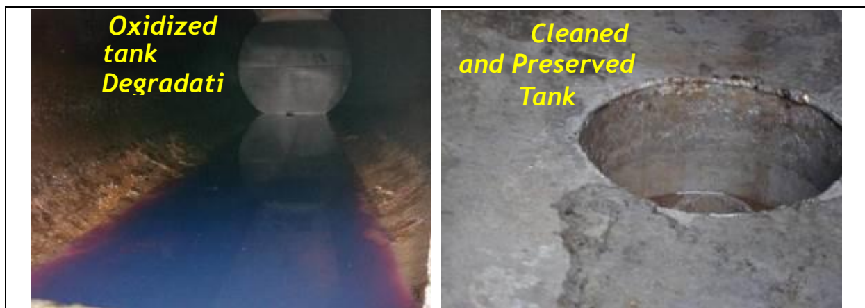
Figure 75 – Oil & Gas – Internal protection of tanks – cleaning process
