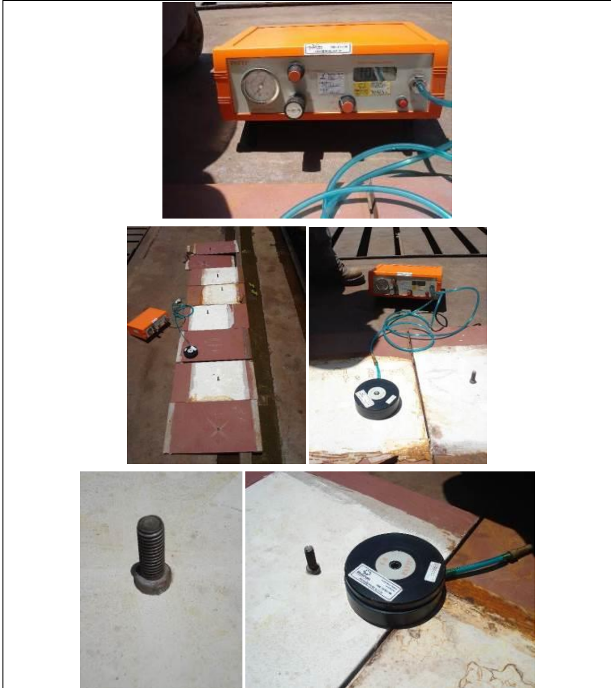
Figure 48 – Steel plates – after hydrojetting – adherence “pull-off” test
