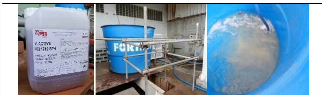
Figure 42 – Preparation of the 10,000L water solution with 2% V-active VCI1712SPH
