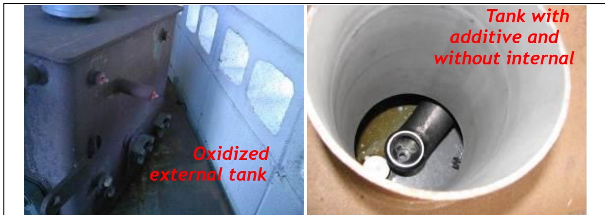
Figure 74 – Oil & Gas – Internal protection of fuel tanks
