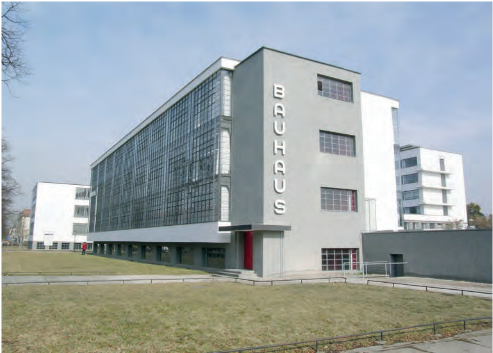
Fig. 1 Bauhaus, southern façade, after conservation. Repair and reconstruction of the plasters and paint, 2006. (Photo T. Danzł)
