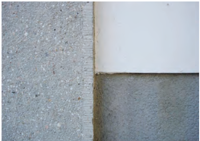
Fig. 4 Bauhaus, repaired and reconstructed façade materials: - lime wash, scratched "Terranova", "Steinputz" treated as artificial stone, 2006. (Photo Danzł)
