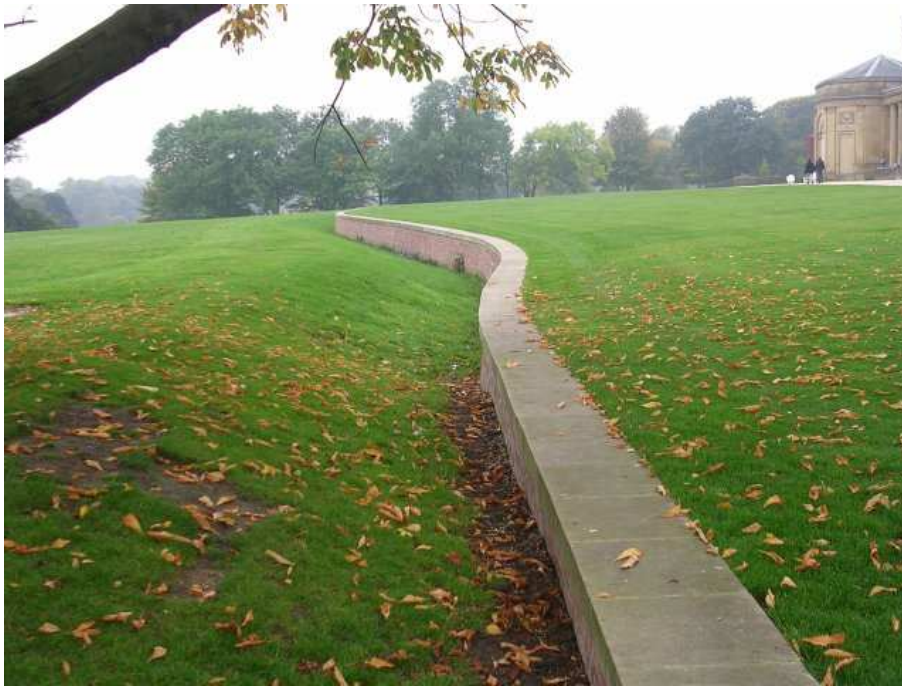
Appendix 1 Heaton Park – a ha-ha wall which opens a park to the surrounding countryside but protects it against animals (photo K. Williams, 2005)
